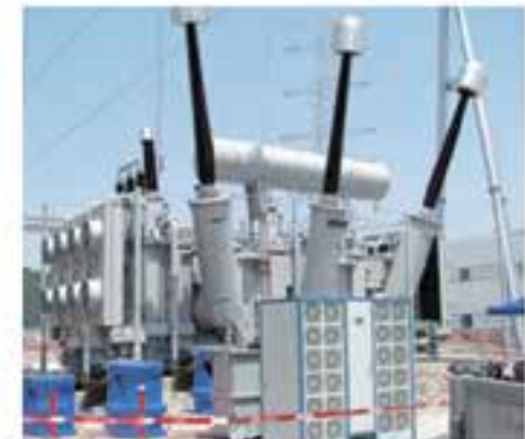
Electro-mechanical inspection offline
